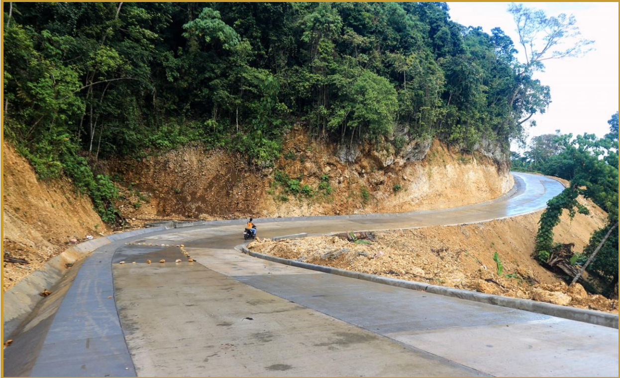
Ongoing Construction of Access Roads Going to Sicalao Falls, Lasam, Cagayan
